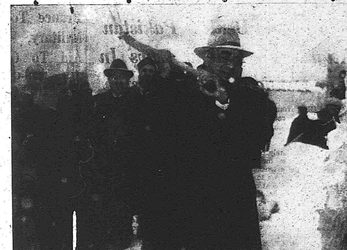
Mayor Asghar officiating the demolition of buildings in the park area when he struck the first pick. (Story on page 1).
